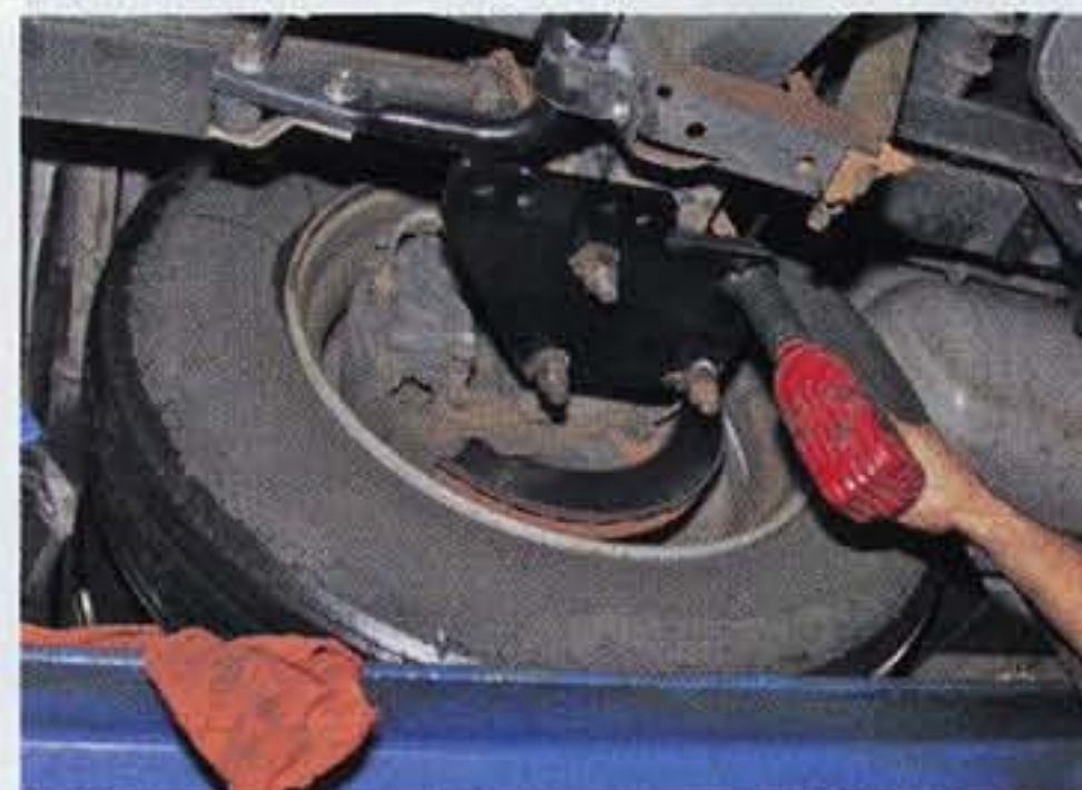
Roadmaster steel brackets are fitted below rear axle, using existing U-bolts.
